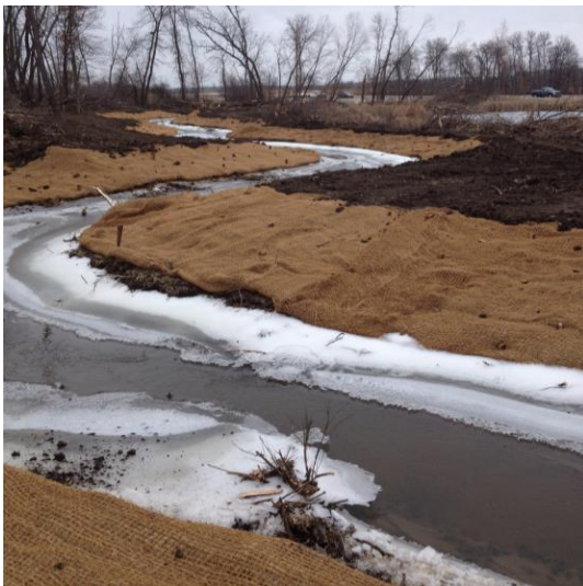
Description. Resloped Banks Constructed During Winter Work on Elm Creek.
