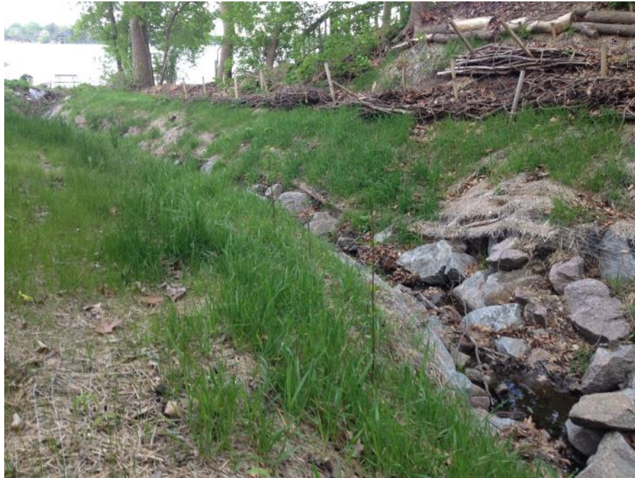
Figure 1: Vegetated Riprap Channel, 1 year after construction.
