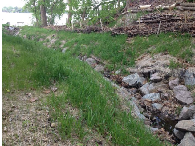
Description. Vegetated Riprap Channel, 1 year after construction.
