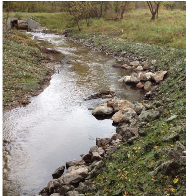
Figure 4: Three stream barbs to turn the flow of Purgatory Creek away from sharp outside bend.
