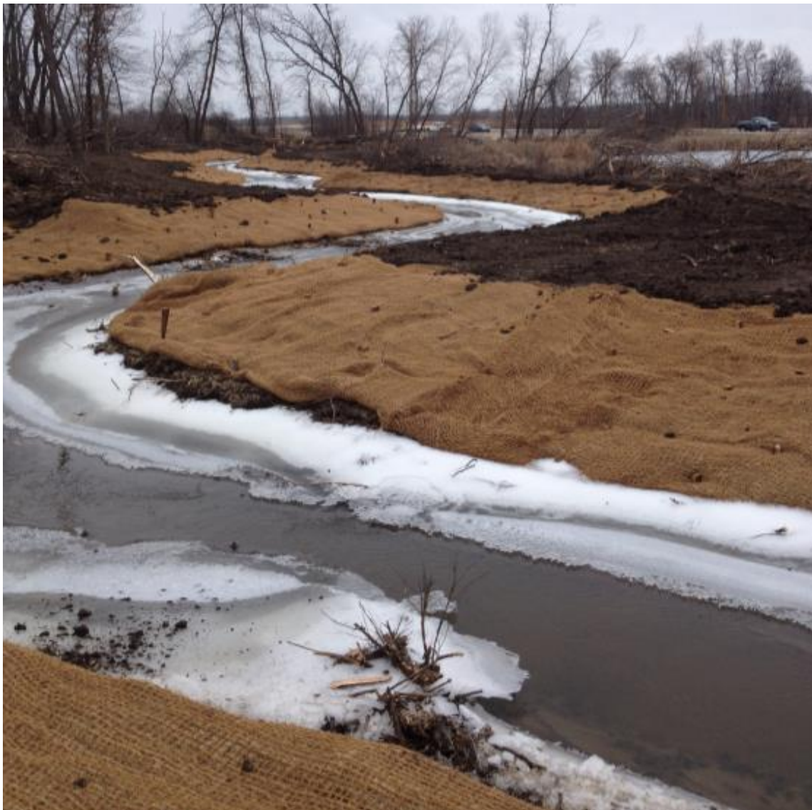
Figure 2: Resloped Banks Constructed During Winter Work on Elm Creek.
