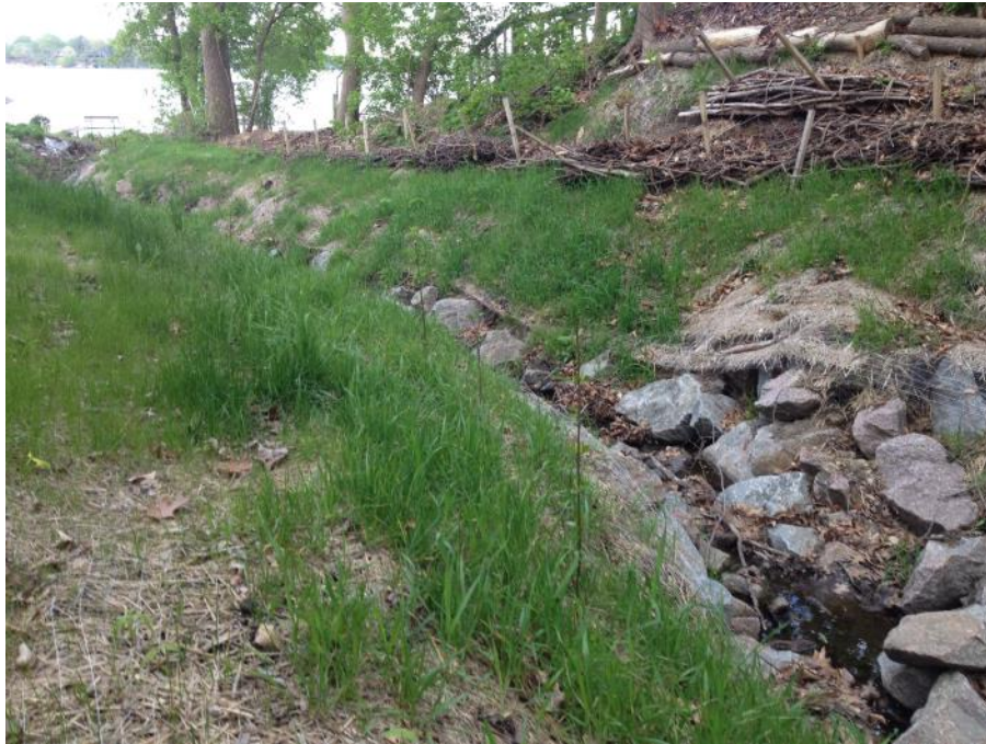
Figure 1: Vegetated Riprap Channel, 1 year after construction.
