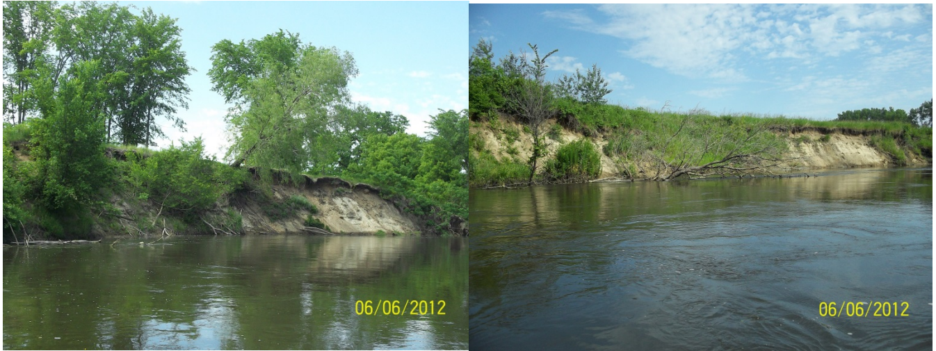
Figures 16 & 17: Significant streambank erosion at Bank #1 and Bank #4 in this reach.
