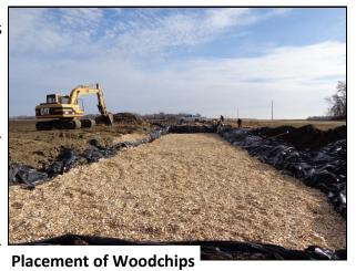
actor can last up to twenty years. Careful management of the water levels in the bioreactor will improve the efficiency of nitrate removal while prolonging its lifespan.
