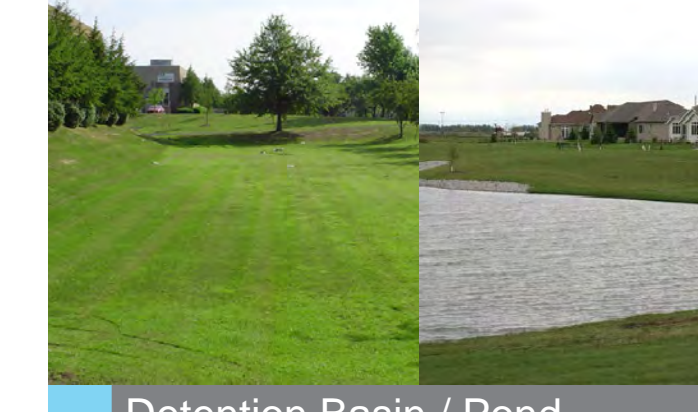
Detention Basin / Pond
