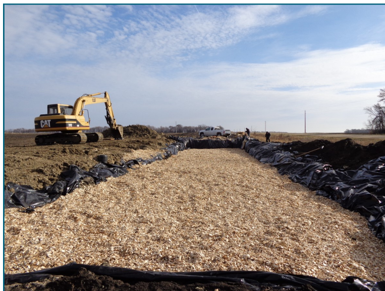
WOODCHIP BIOREACTOR INSTALLATION
