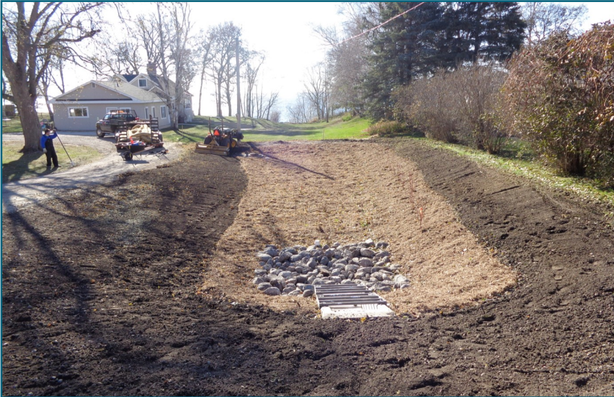
INFILTRATION BASIN ON IRVING TOWNSHIP PROPERTY
